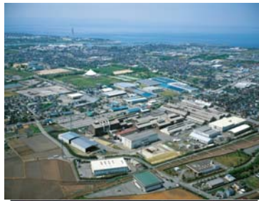
Higashi-Toyama, Steel Plant
